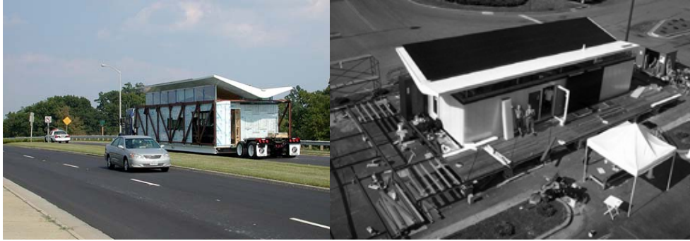
Figures 8 and 9. Initial testing of transport structure; final stages of assembly.
